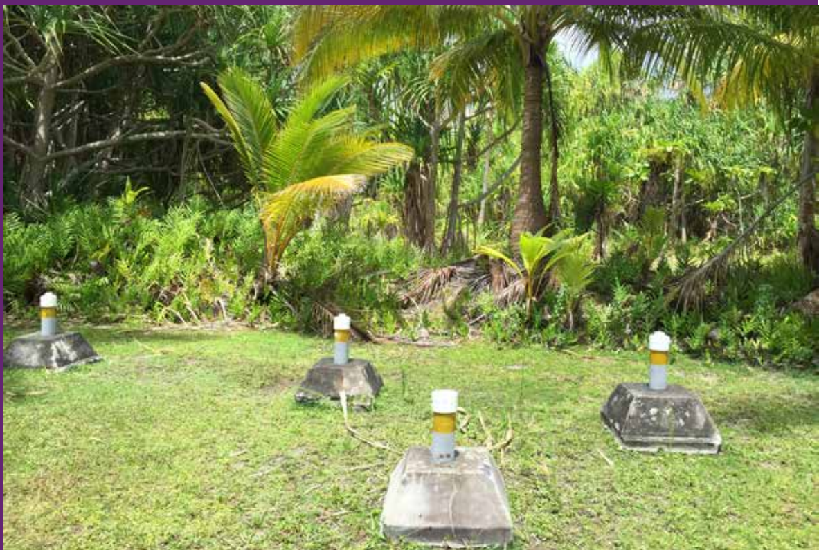
Groundwater monitoring wells on Roi-Namur Island, Kwajalein Atoll, Republic of the Marshall Islands.
