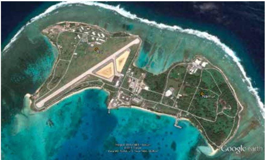
Two concrete-lined rainwater catchment basins on Roi (visible on image to left) are used to collect rainwater and artificially recharge groundwater when there is excess capacity Sources : Google Earth
