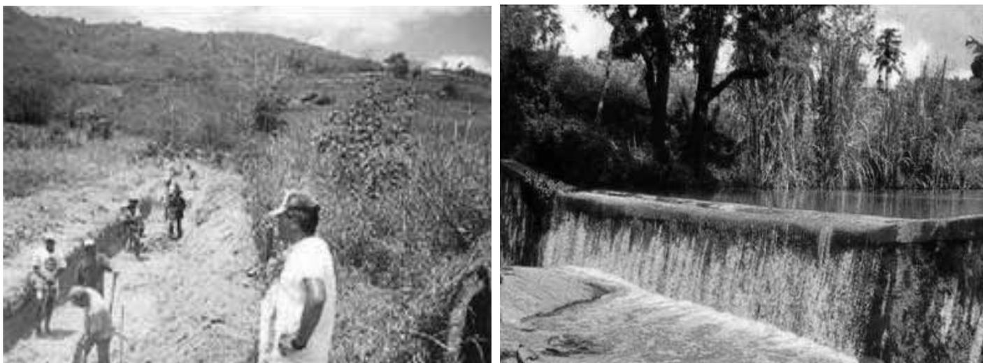
The storage capacity of a typical subsurface dam and reservoir (say in average of 4 m depth, 50 m width and 500 m length) will be some 10,000 m<sup>3</sup>, assuming a drainable storage coefficient of 0.10. This is not sufficient for these dams to provide multi-annual regulation, unless their usage is only for human and animal consumption. However, intra-annual regulation makes possible the use of water for small-scale irrigation in the dry season, enabling the production of various crops.
