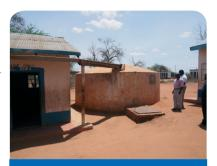
3R example: Rain water harvesting tank, collecting water during the rains from rooftops and storing it in tanks provides a source of good quality water.
