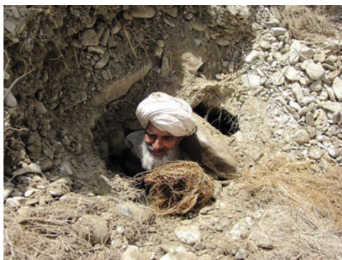
Figure 20. A specialized Karez cleaner in Qila Iskan Khan, seen with a dot of grass removed from the underground canal bed. Due to the high risks involved and the special skills required, it is a well-paid job (Photo: IUCN Pakistan, 2010).
