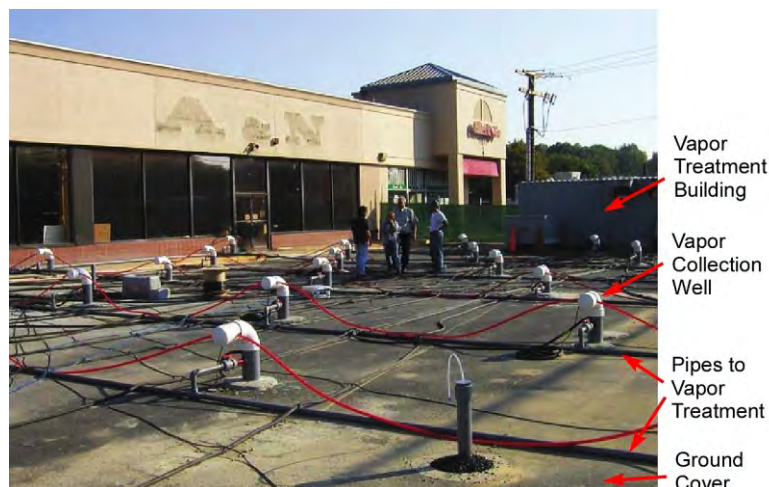
Figure 13.23 ERH system for remediation of contaminated soil and groundwater. Note that the surface was paved to prevent cooling effects of aerial recharge. From EPA-542-F-21-016, in public domain.
