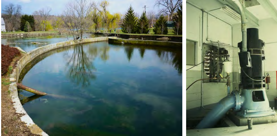
Figure 16.39 Left: Abandoned capture of a spring historically used for public water supply of Winchester, Virginia. Right: Pump house at a large spring utilized for public water supply of a township in one of the central U.S. states. The spring is one of the most productive in the state, supplying about 5 million gallons of water per day for domestic and municipal use.
