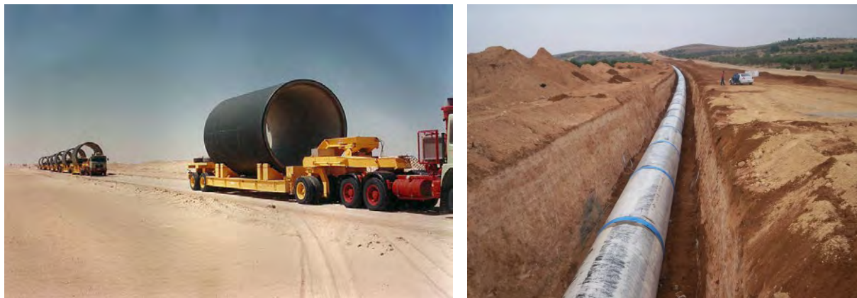
Figure 16.17 For the construction of Great Man-Made River project in Libya, prestressed concrete cylinder pipes 4 meters in diameter and 7.5 meters long, weighing up to 80 tons, were brought to the excavation sites using a fleet of some 128 specially designed transporters. Each pipe was buried in a trench approximately seven meters deep, excavation of which required the removal of some 100,000 cubic meters of material each working day. Excavation was carried out by large hydraulic excavators fitted with 7.6 m 3 buckets. Left photo courtesy of Jaap Berk, The Netherlands; in public domain. Right photo courtesy of https://alk3r.wordpress.com/2017/07/04/the-great-man-made-river-of-libya/ .
