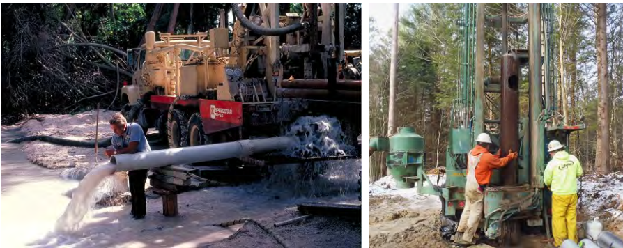
Figure 16.24 Well development methods. Left : Airlift, photo courtesy of Dr. Gerald Seaburn. Right : Bailer, photo courtesy of Mark Bauer.
