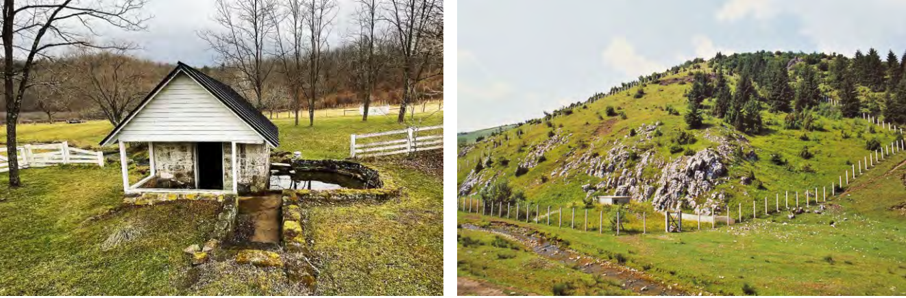
Figure 16.37 Left : Spring house built on top of an ascending spring at a historic plantation in Bath County, Virginia. The house also served as a food storage because of the cool air maintained by the spring water. Right : Spring-box type capture of the Lakomica spring issuing at the contact between fractured limestone and underlying low-permeable diabase. Fence around the spring area prevents access to the capture. The spring supplies drinking water to a town in western Serbia.
