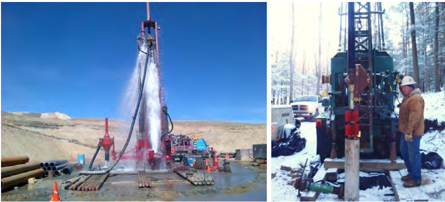
Figure 16.23 Well development methods. Left : Compressed air, photo courtesy of Dave Evans. Right : Wire brush, photo courtesy of Mark Bauer.
