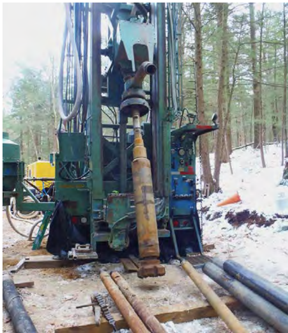
Figure 14.23 Rotary drill bit on a dual rotary drill rig used to install a monitoring well in a karst aquifer in New York state, United States. Courtesy of Mark Bauer.
