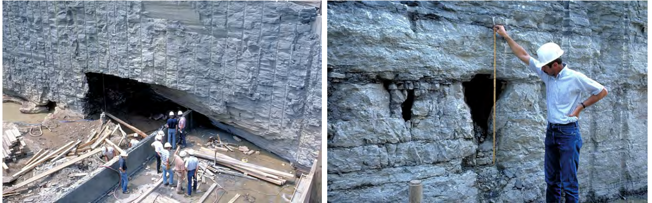
Figure 7.15 Cavities of varying size discovered at a deep (seen dewatered here) construction site in Hartsville, Tennessee. Photographs by George Sowers; printed with kind permission of Francis Sowers.
