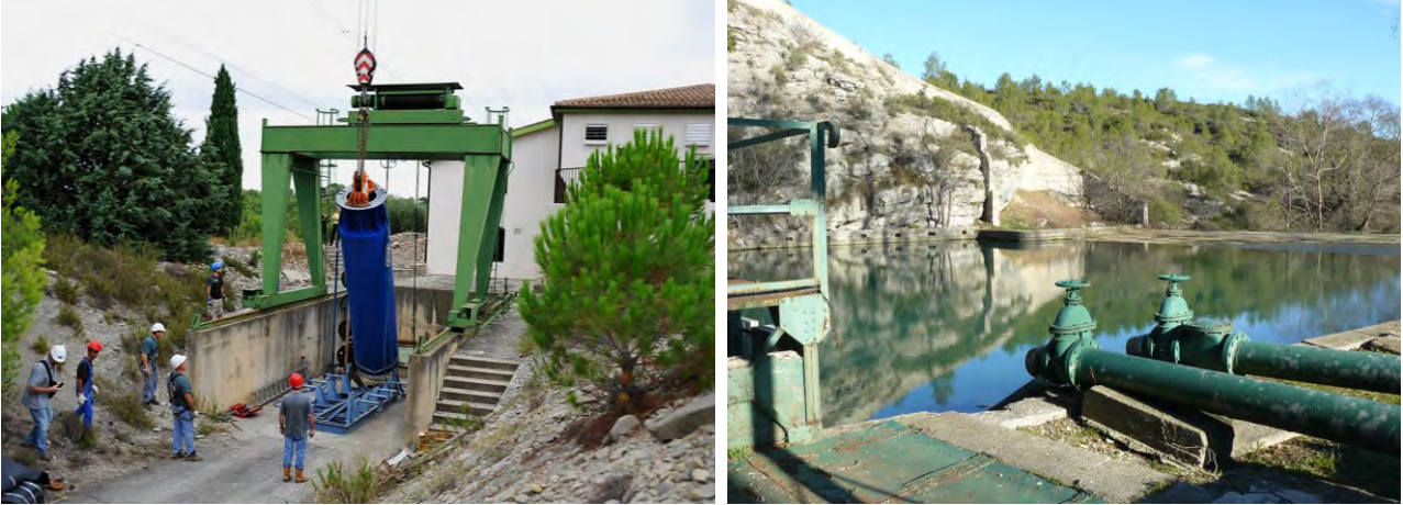
Figure 16.43 Left : Replacement of a high-capacity submersible pump in one of the extraction wells at the Source of River Lez (Source du Lez) utilized for water supply of Montpellier, France. Photo courtesy of Jean Michel Valéry. Right : Old pumping installation at the spring. Photo courtesy of Arnaud Vestier, Service des Eaux, city of Montpellier.
