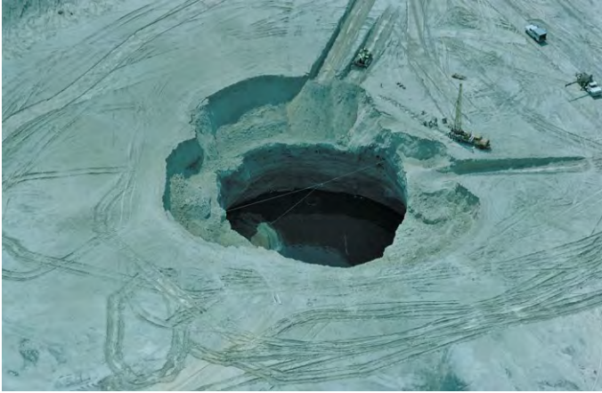
Figure 12.4 A gaping sinkhole formed abruptly on June 27, 1994, within a 400-acre, 220-ft high gypsum stack at a phosphate mine in south-central Florida. Note trucks and the drilling rig for scale. Photo by late Professor George Sowers, printed with kind permission of Francis Sowers.
