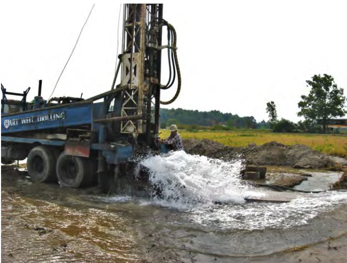
Figure 6.23 Development of a high yielding well in Michigan, completed in glacial sand and gravel aquifer. Photo courtesy of Jim Brode.
