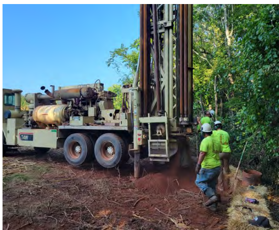
Figure 14.24 Air rotary drilling during a monitoring well installation at a coal ash landfill in Eastern United States. Courtesy of Ted Wilson.
