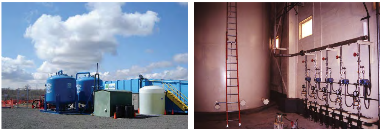
Figure 13.16 Left: Outdoor treatment facilities. From EPA-542-F-21-021. In public domain. Right: Control room for a P&T system with five extraction wells; extracted groundwater treatment tank is on the left.
