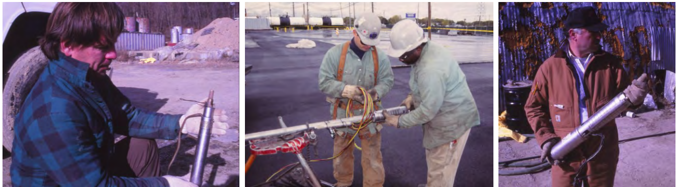
Figure 16.26 Submersible well pumps come in many different sizes and capacity, from gallons per minute to tens of gallons per minute (shown on the photos), and as powerful as hundreds of gallons per minute or more, with the lift of hundreds of feet or more.
