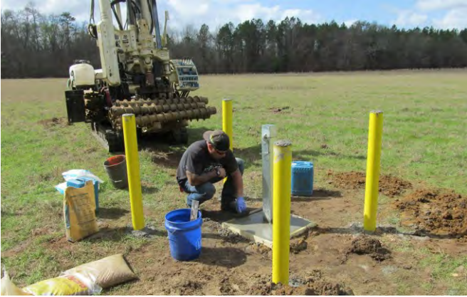
Figure 14.27 Typical completion of a monitoring well showing riser pipe, concrete surface pad, and bumper guards for surface protection. Hollow stem auger drill rig is in the background. Photo courtesy of Dawit Yifru.
