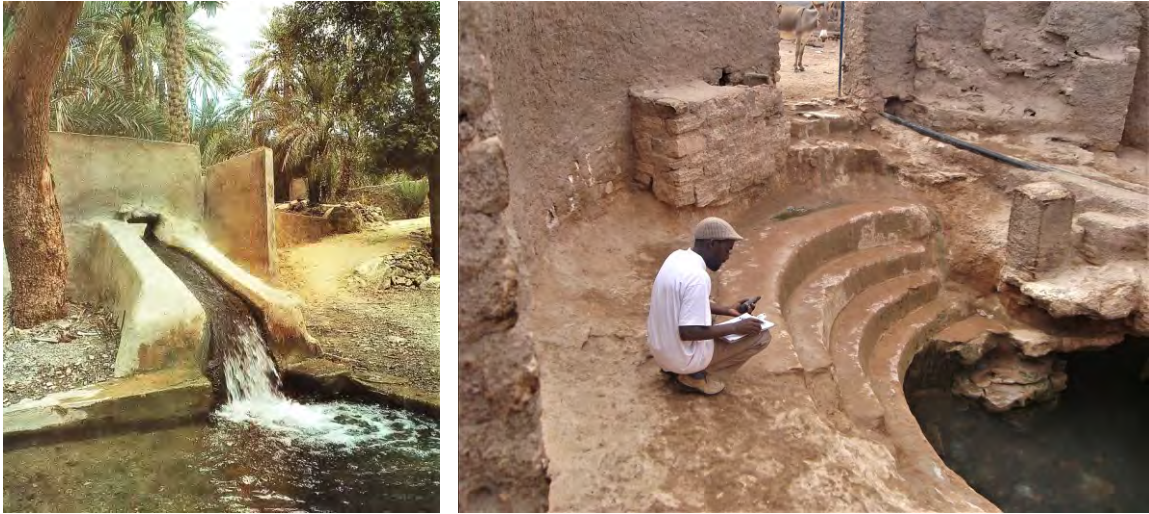
Figure 16.34 Left : Capture of Hammam Sharqi Spring in the Sultanate of Oman. Part of water (seen here) from this hot spring ( 41^{\circ}\text{C} ) is used for irrigation. Chebaane et. al (1994). Right : Ancient spring intake Taalex Laasqoray Xudun, still actively used by local population; Sool Plateau-Sanaag, Puntland Province, Somalia. Courtesy of Zoran Stevanović.
