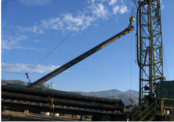
Figure 16.19 Large-diameter casing being installed in a deep production well in Arizona. Photo courtesy of Adrian Ezeagy.
